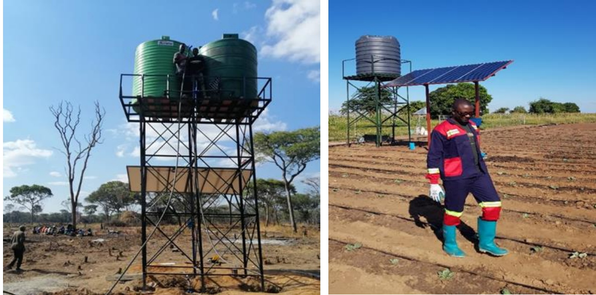
Figure 9: Irrigation system in Zambia (left) and Zimbabwe (right), using water from the borehole.
