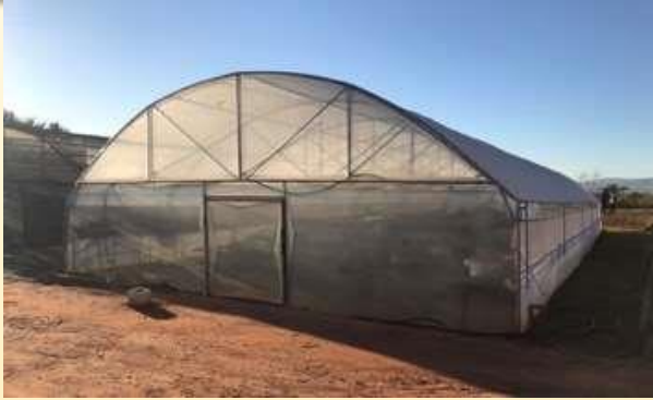
Rebuild a Greenhouse
